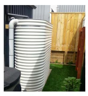
The Detention Tank works by temporarily storing the collected rainwater and then slowly releasing the water through a small outlet in the tank. This storage and slow release of the rainwater reduces the peak stormwater flows during a rainfall event and hence reduces the impacts on downstream infrastructure and/or streams.
